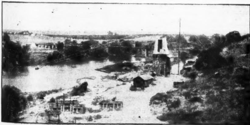
Views of Service Brothers Plant
